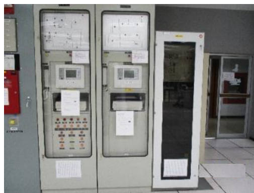
Slave Fire Alarm Panel
