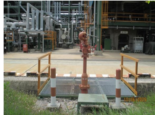
Water Hydrant with Monitor
